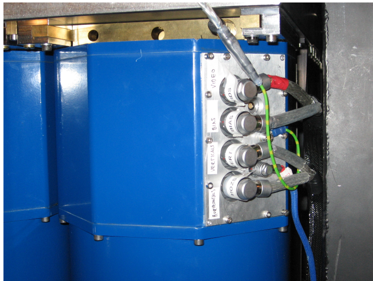
Figure 6: Detector connector panel showing CCD cables installed. The grounding plug is the yellow-green wire.
